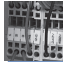
Provided terminal blocks allow for connection to remote Start/Stop station.
